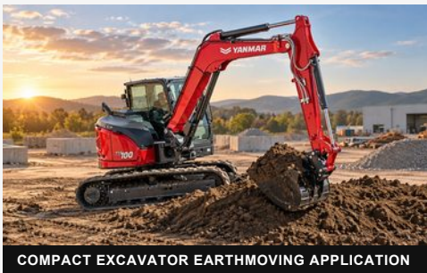
COMPACT EXCAVATOR EARTHMOVING APPLICATION
