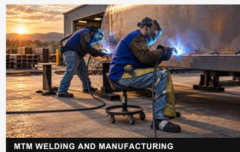
MTM WELDING AND MANUFACTURING
