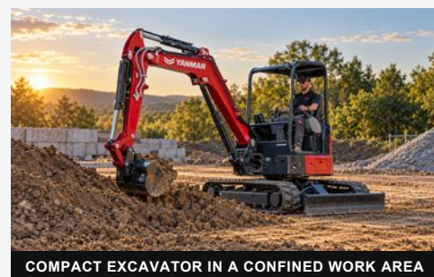
COMPACT EXCAVATOR IN A CONFINED WORK AREA
