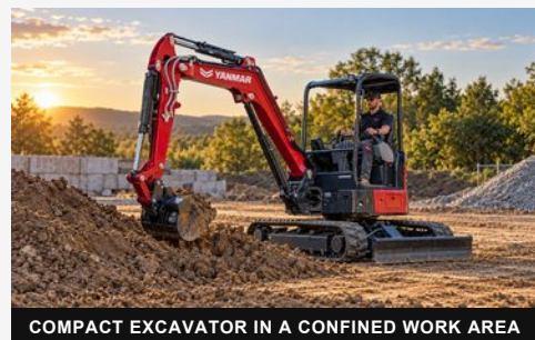
COMPACT EXCAVATOR IN A CONFINED WORK AREA
